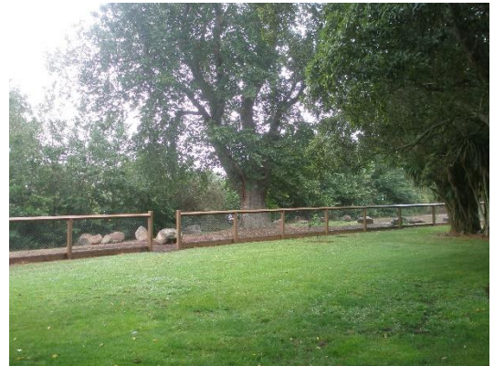
An approximately 110–120cm high timber (posts, top rail, gravel board) and cyclone wire fence defines the boundary of the Botanic Gardens. This fence replaced an earlier fence in 2004–05, reported to have been ‘dilapidated’. 191
