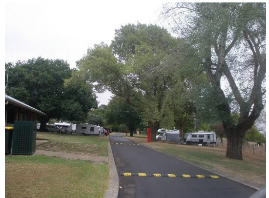
Section of bituminised road within the caravan park, with kerbing and speed humps.
