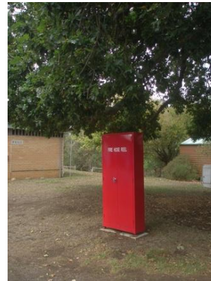
One of the services (fire hose reel) associated with caravan park, installed to meet compliance requirements, in 2013.
