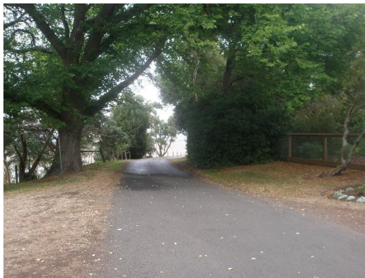
Section of bituminised road which leads to the lookout (immediate south of the Gardens enclosure) with no kerb.
