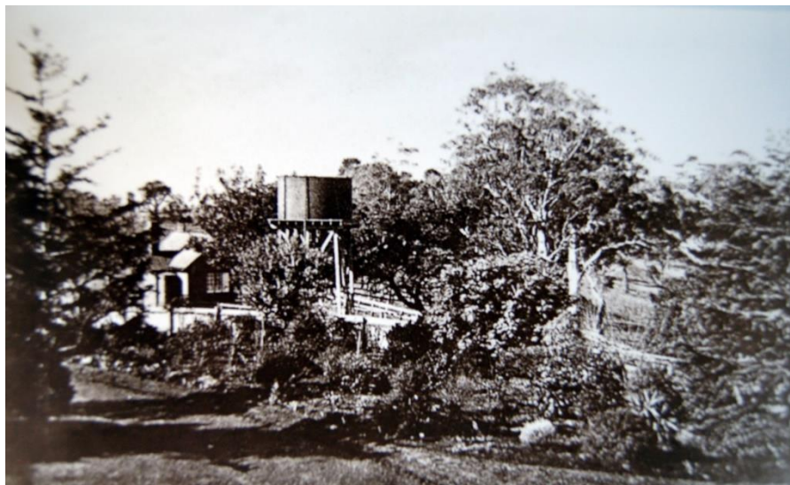
Image of shelter (probably the kiosk) and adjacent water tank located outside entrance gates, photographed from within the enclosure, c.1910s. Water boiled at the fireplace no doubt was collected by the adjacent water tank on timber tankstand. (source: CDHS)
