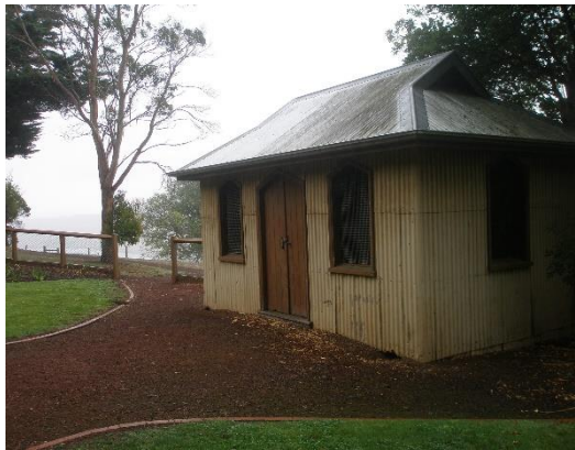
Pedestrian entry to the Gardens enclosure, near the iron Potting Shed (Feb 2016)
