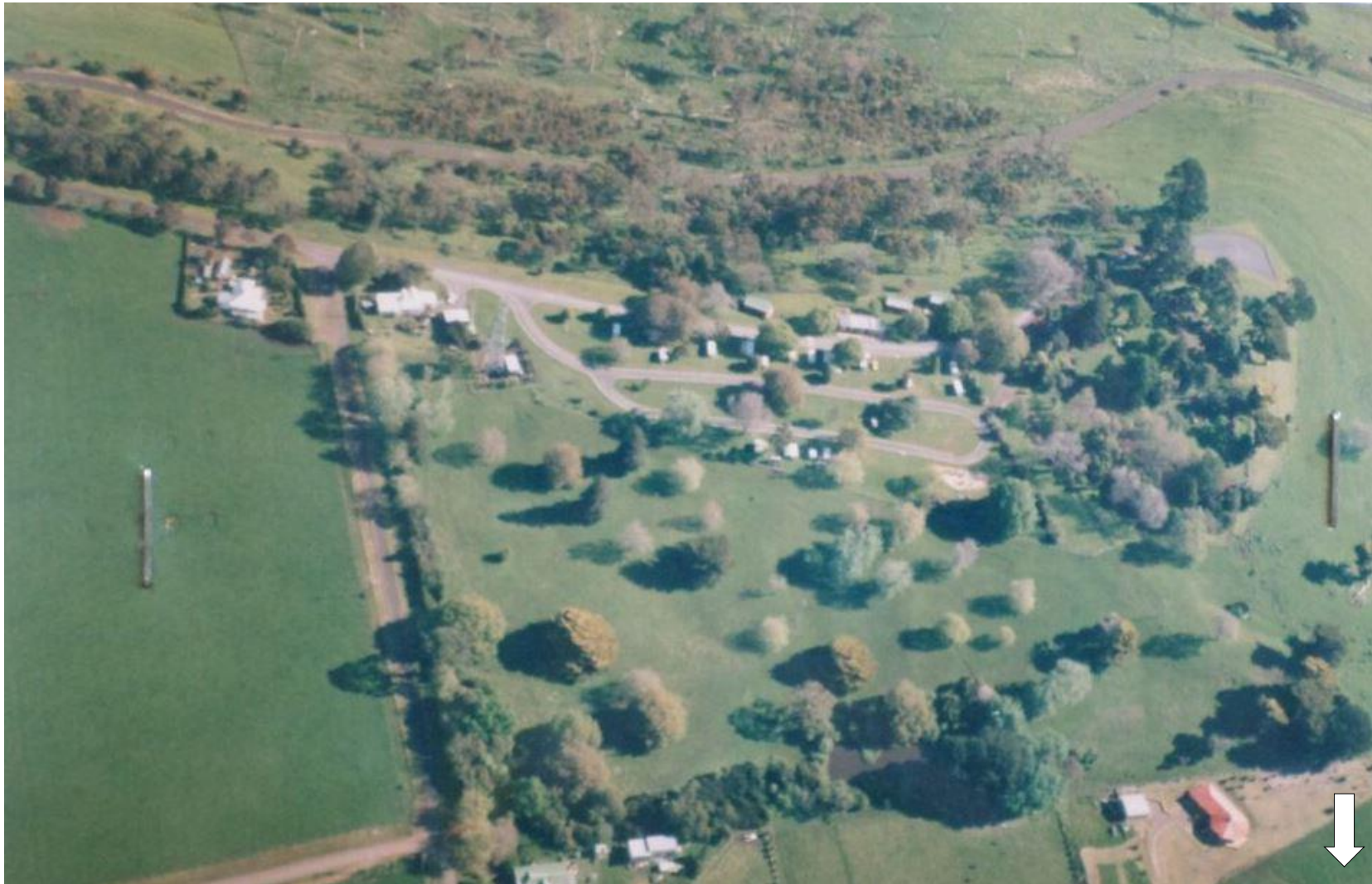
c.1984: Oblique aerial view of eastern part of study area, looking south (source: Rs file 3586, DELWP). Approximate north indicated by arrow.
