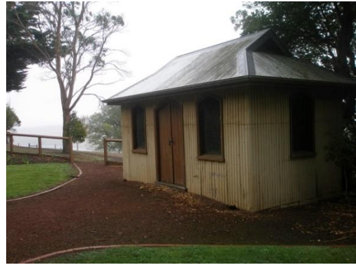
The Potting Shed at the western edge of the Gardens in February 2016.
