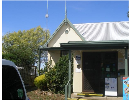
Steep-pitch roof and prominent gable remnants of the late nineteenth century caretaker's cottage.
