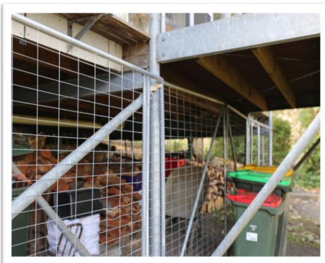
Figure 31 Heavy fuel stored under a house
