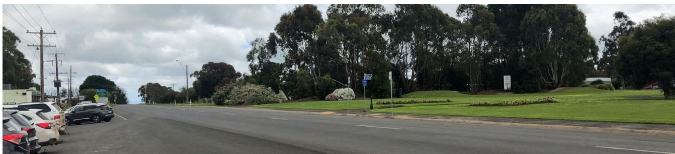
Image 11. Lavers Hill-Cobden Road adjacent to Jaycees Park
