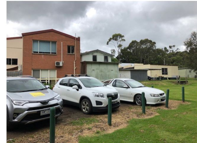
Image 5. Interface with Powers Creek valley (back of buildings facing Main Street).
