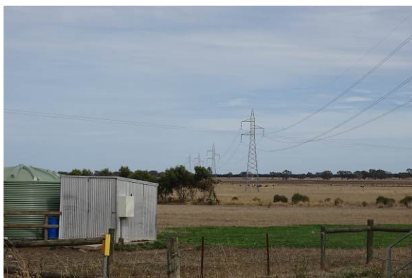
I: Power lines and farm related structures (view from Darlington Rd towards the Site)
