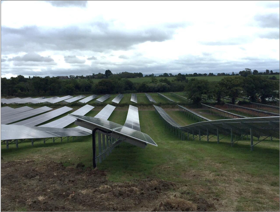
Figure 3: Fully assembled fixed array solar far (image supplied by Infinergy UK)
