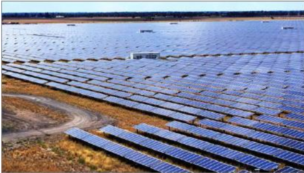
A large scale solar farm using a tracking system
