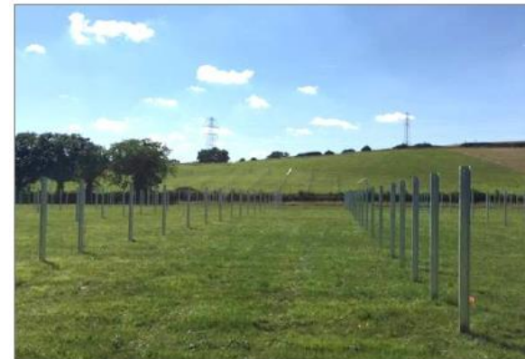
Example of piles during the construction of a solar farm
