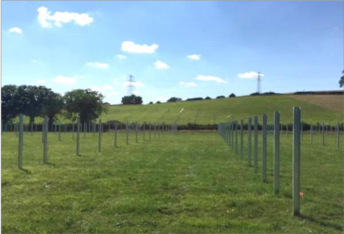
Figure 1: Piles for a solar farm in place (image supplied by Infinergy UK)
