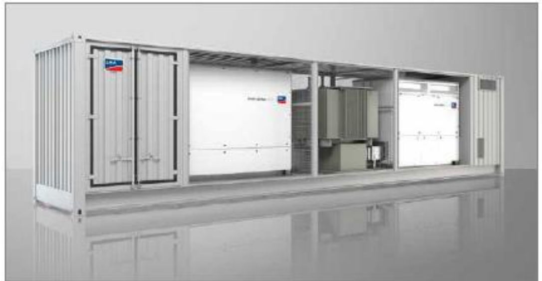
A containerised inverter
