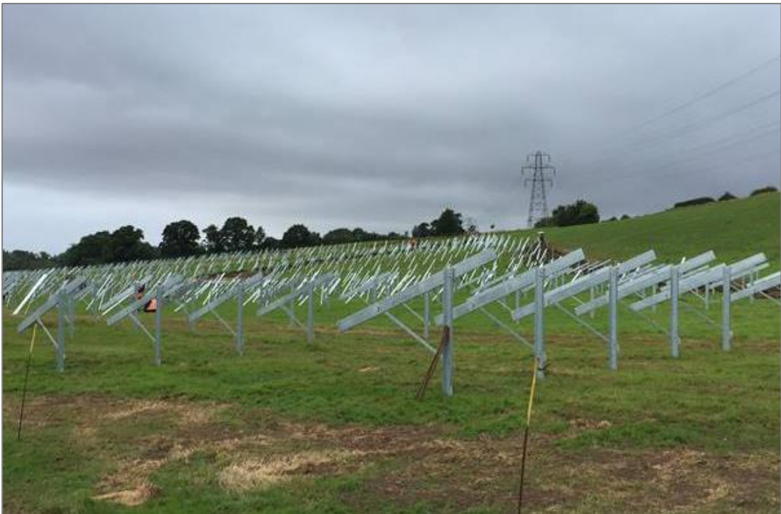
Figure 2: Fixed array assembled before PV panels added (image supplied by Infinergy UK)
