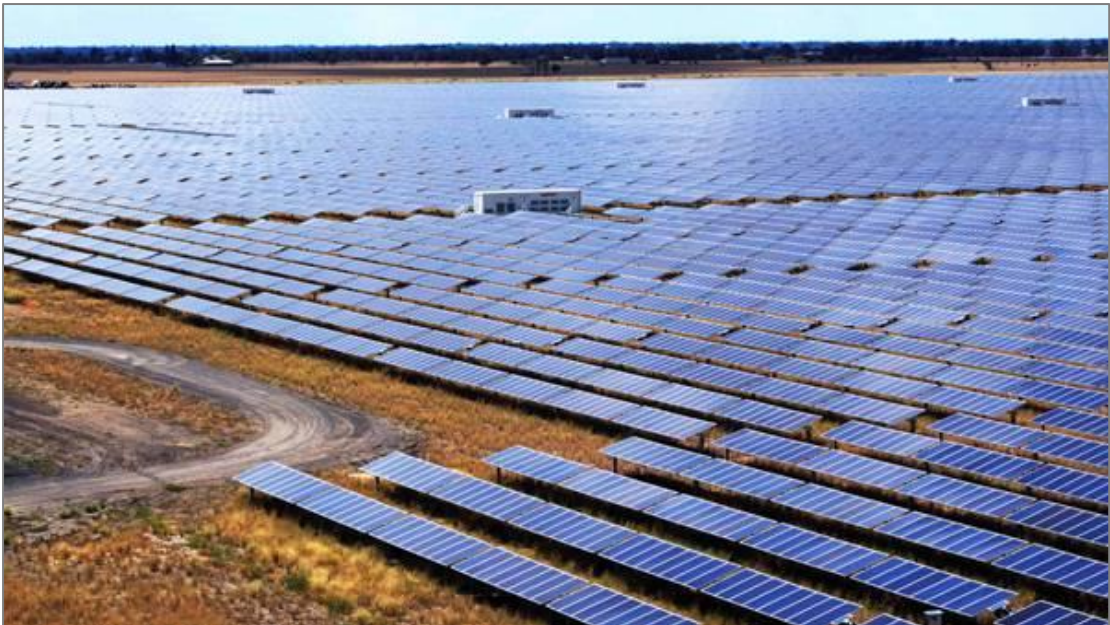
Figure 4: Fully assembled tracking array solar farm showing inverter housing (image courtesy Nexttracker Australia, actual tracking system and inverters may differ). At solar noon panels face directly upwards. In the evening they face 60 degrees to the west and vice versa in the morning.
