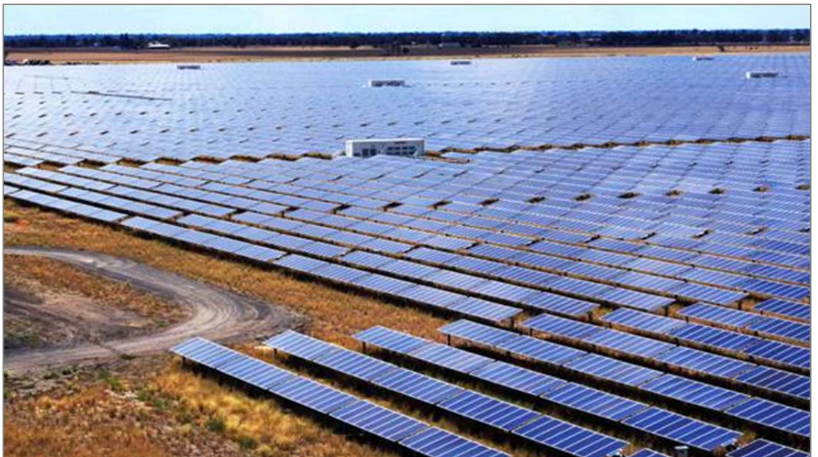
Figure 4 – Example of a fully assembled tracking array solar farm showing inverter housing (Source: Nextracker Australia).
