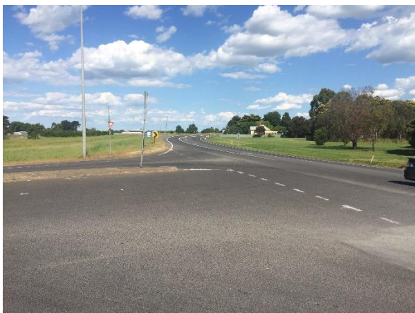
Princes Highway looking east
