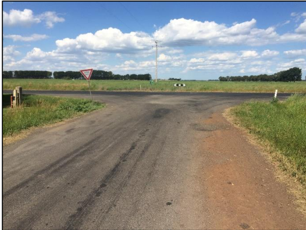
Blind Creek Road looking east
