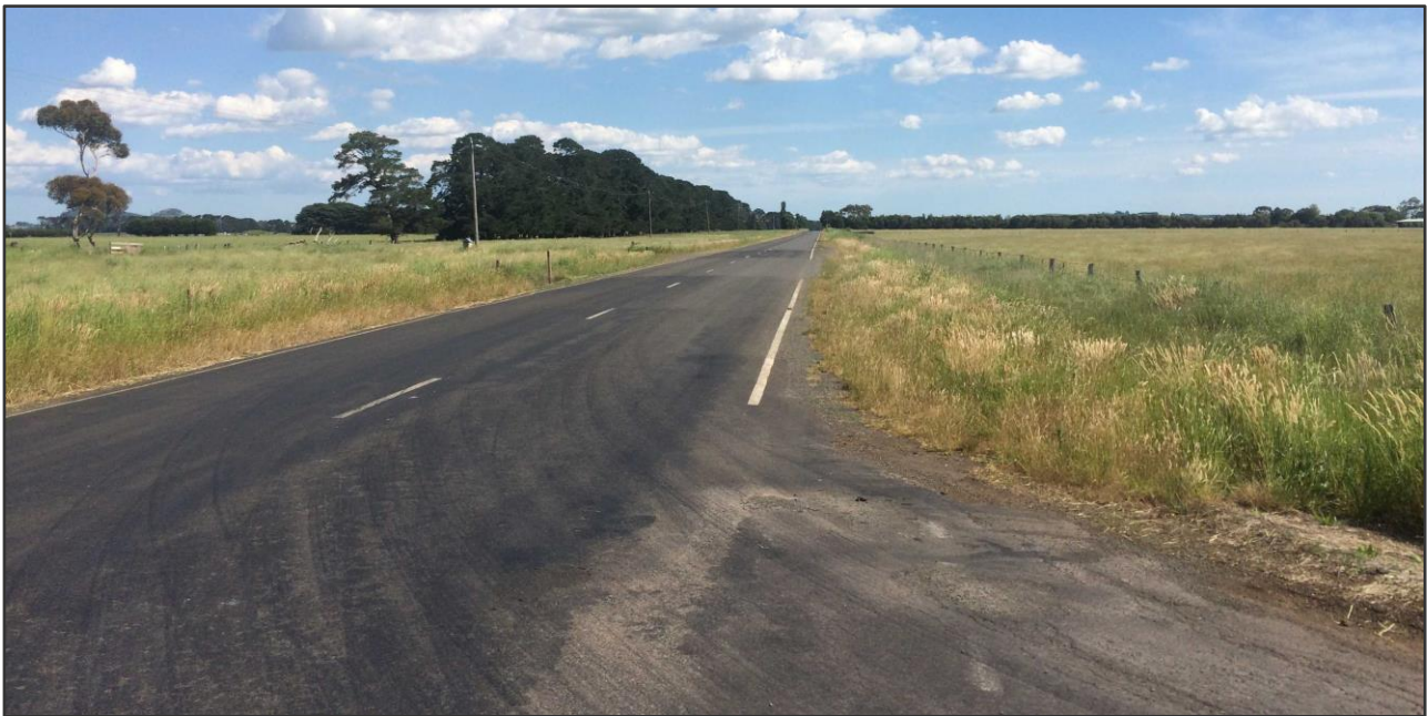
Figure 3 Darlington-Camperdown Road, looking south from Blind Creek Road
