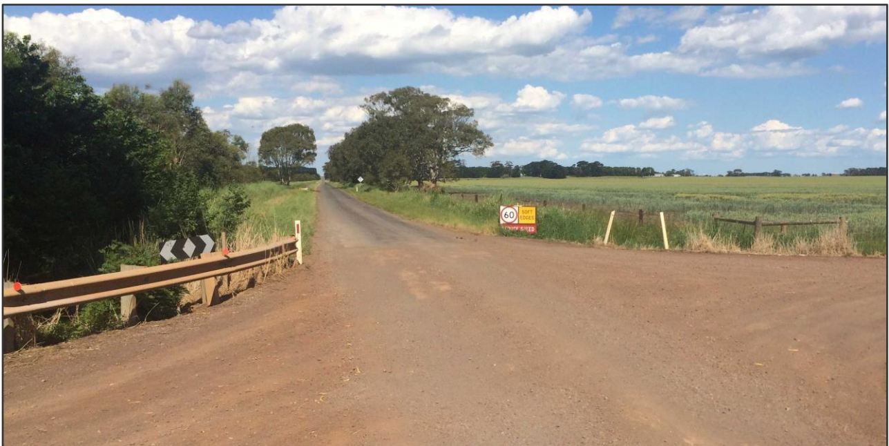
Figure 4 Blind Creek Road looking east from Meningoort Road
