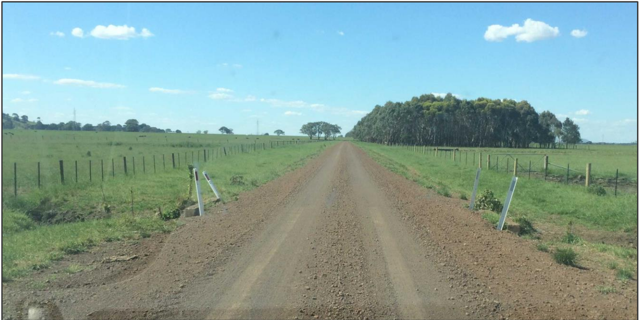
Figure 5 Meningoort Road, looking north with the existing culvert
