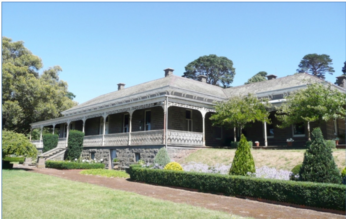
Figure 2: Meningoort Homestead Front Porch, Victorian Heritage Database 2008.
