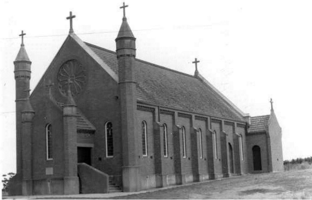
St Joseph's Catholic Church, Noorat, designed in 1919 by Melbourne architect Bart Moriarty [SLV]
