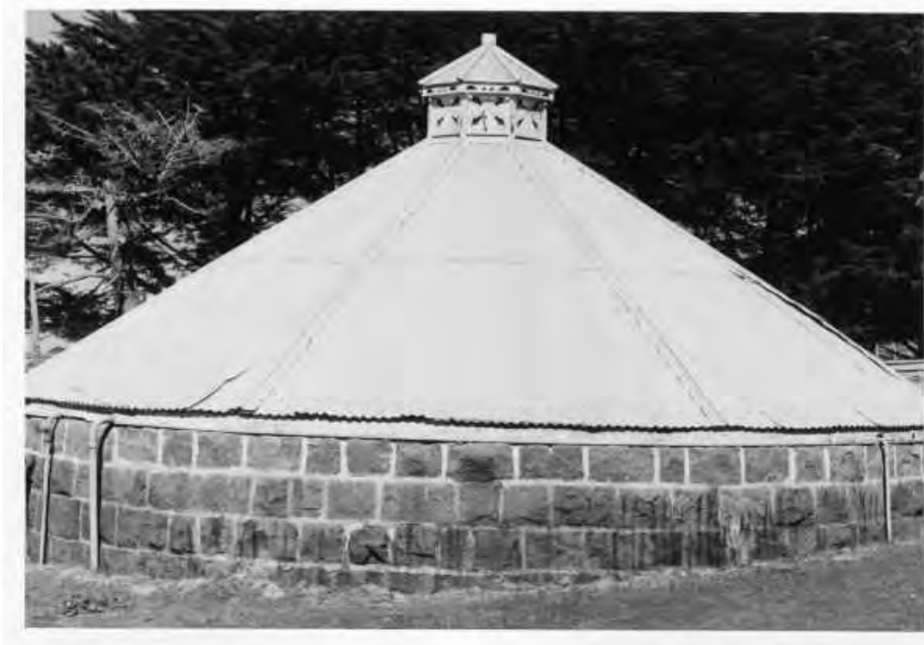
Bluestone tank at Talindert, near Camperdown, probably c.1870s [SLV]
