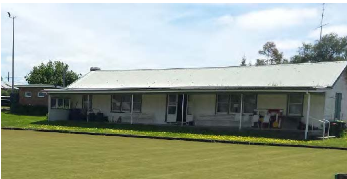
Figure 1: The Club House, 30 – 32 William Street, Lismore
