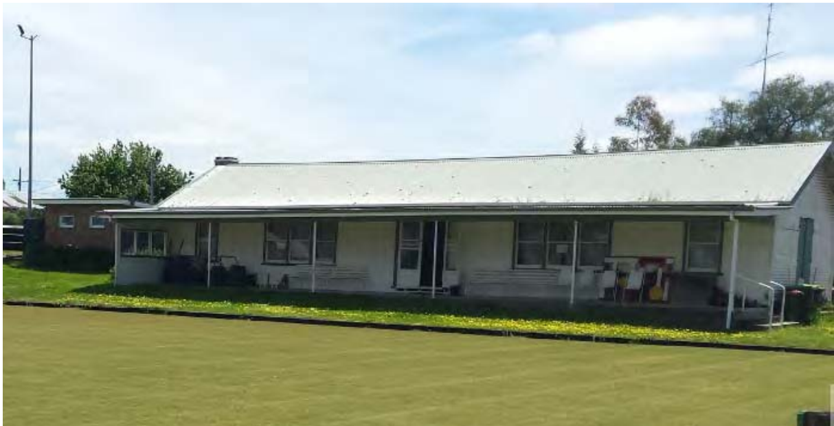
Figure 1: The Club House, 30 – 32 William Street, Lismore
