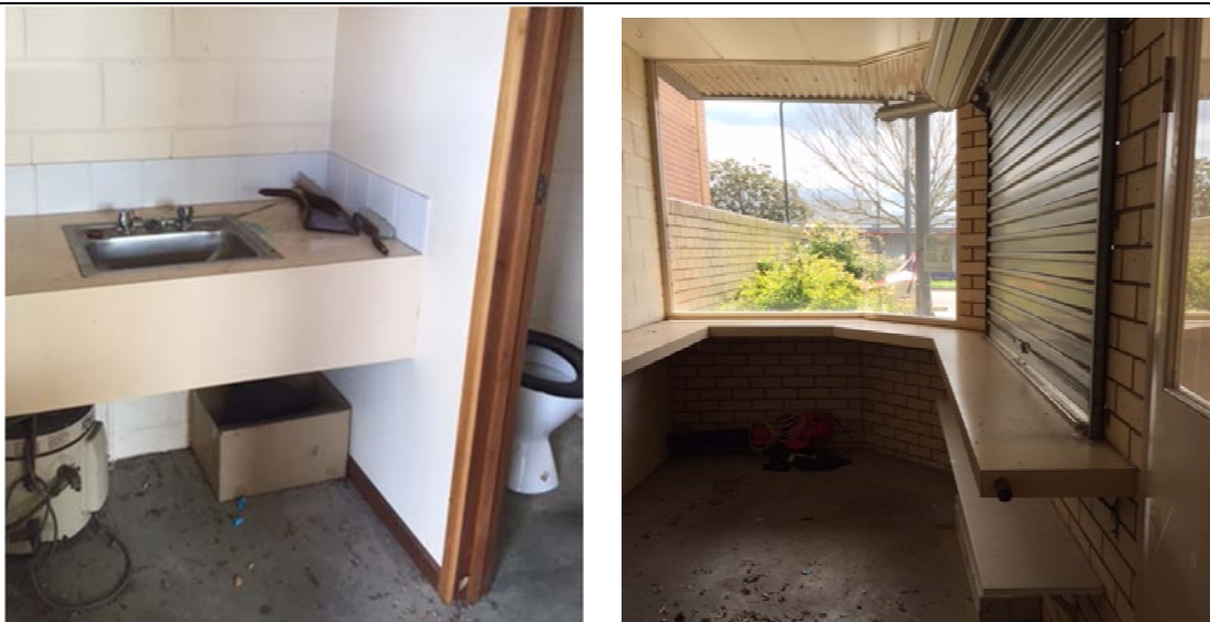
Figure 3 & 4: Internal Photo of 19F Curdie Street, Cobden
