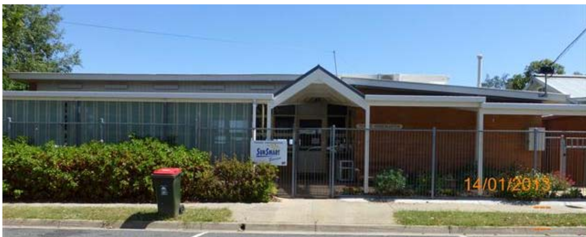
Figure 1: Former Terang Kindergarten, The Promenade, Terang
